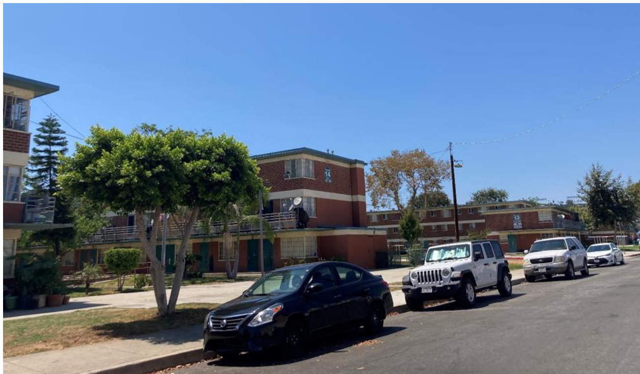
Figure 4.1-6 Leroy Street and Bolero Lane – William Mead Homes
