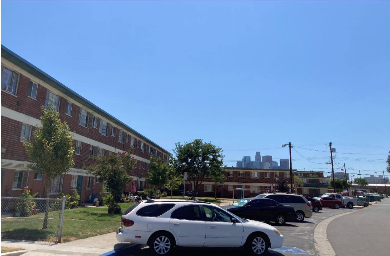
Figure 4.1-7 Leroy Street and Cardinal Street – William Mead Homes
