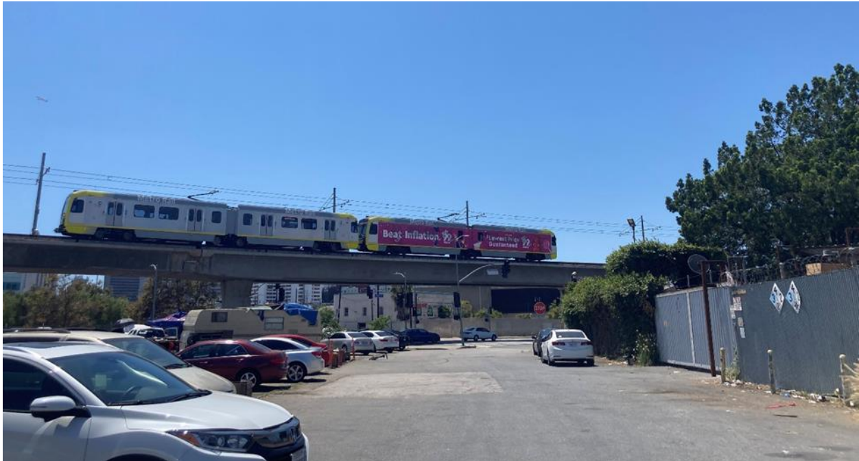
Figure 4.1-2 North Alhambra Avenue - Metro Gold Line in the Background
